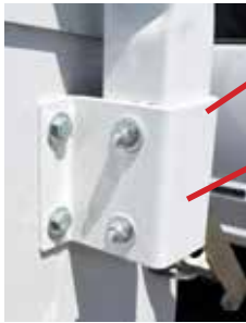
Ladder Rack Bolts
